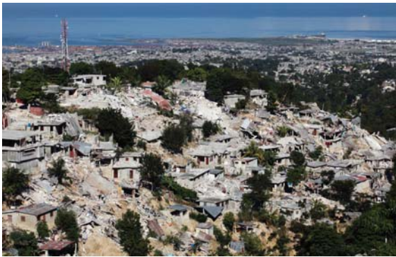
Figure 4. The dire situation in Haiti after the earthquake. Note extensive collapse of nonengineered buildings mimicking a landslide because the buildings are mostly instable when on a slope.
