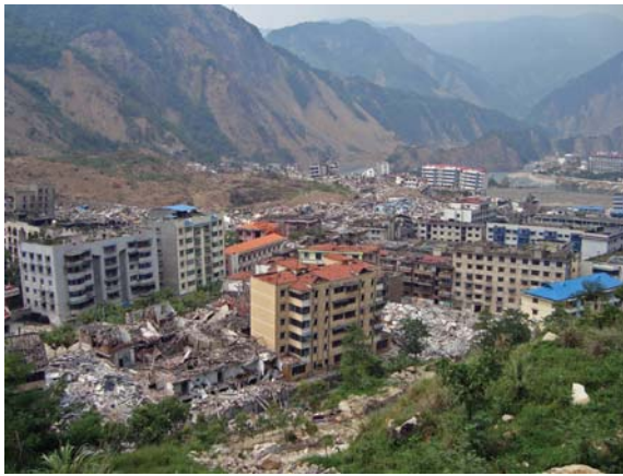
Figure 8. The destruction after the earthquake in Sichuan valley. Note the newer more recently constructed engineered buildings held-up whilst the older poorly engineered ones crumbled. Closer view reveals the crumbling of wood and brick construction but no damage to engineered structure in background. Note building in the center, uprooted from its foundation and toppled.
