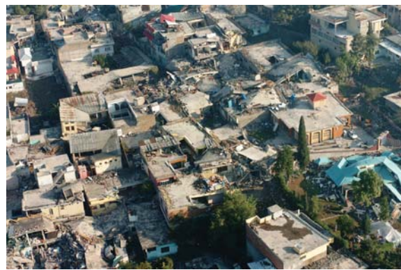
Figure 10. The destruction after the earthquake in Pakistan shows extensively collapsed rooftops due to weak construction of supporting joints.
